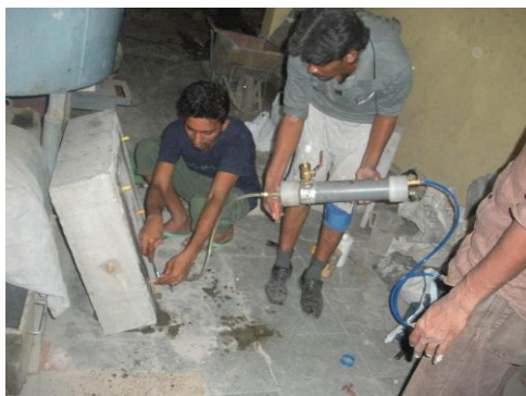
Fig 1. Injection grouting in a slab
